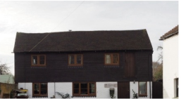
Weatherboarding on first floor
