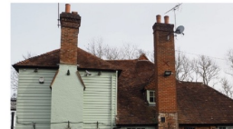
Chimney on the side
