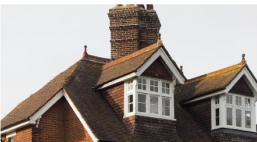
Hipped roof with Kentish peg tiles
