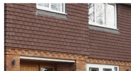
Tiles hanging on the facade (first floor)
