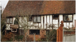
Timber frames with render infills
