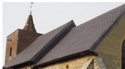
Gable roof with grey slates
