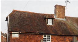
Clipped gable roof
