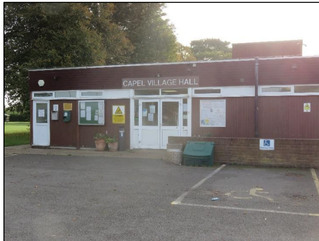
Capel Village Hall, located in Five Oak Green
