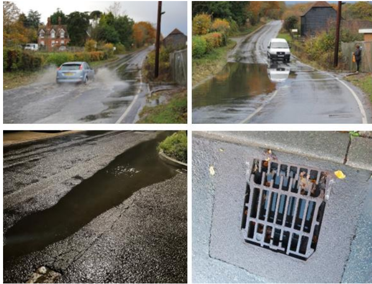
Images show examples of excess water on the roads due to blocked drains and lack of drain capacity
